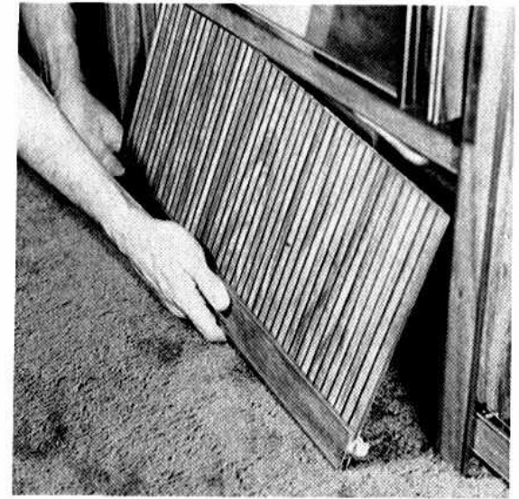
Removing Furnace Access Door
